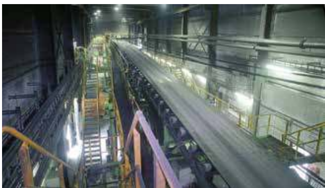
Conveyor belt system
