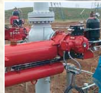
Bladder Accumulator with special coating used for valve actuation. (photo courtesy ROTORK)
