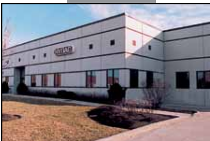
Glendale Heights, IL - Cooling Systems
